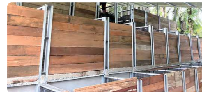
Three-stage composting facility
