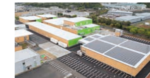
Kanto pharmaceutical factory completed on April 18, 2023
