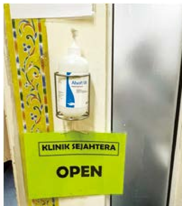
Alsoft A installed on a wall bracket at the clinic's entrance
